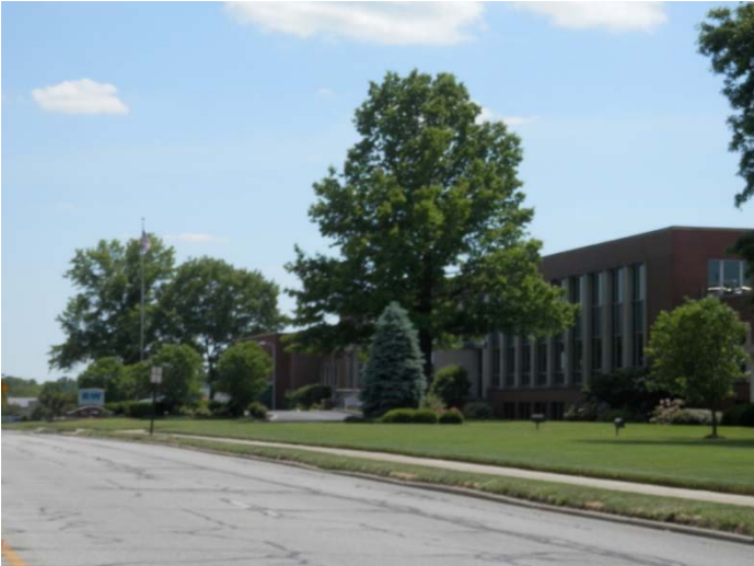
Below: Babcock & Wilcox on Van Buren St looking south
