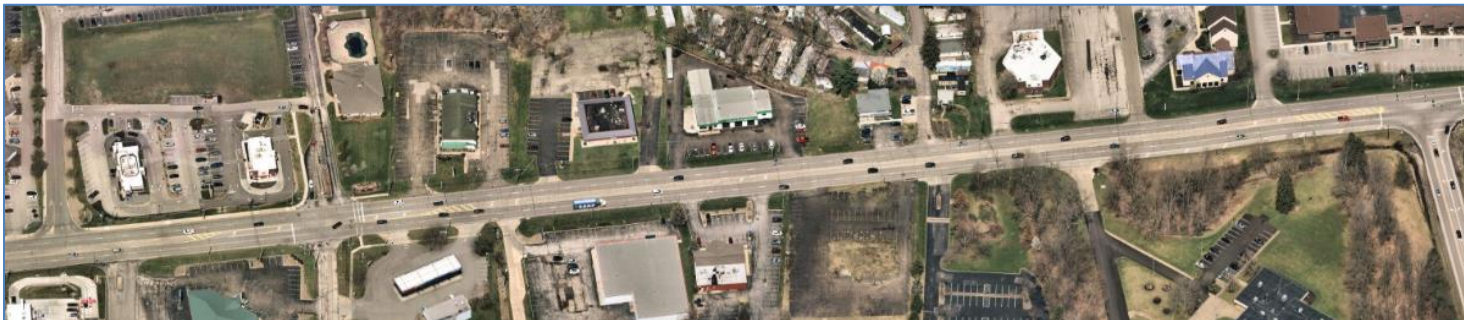
Two sections of SR 59 rank in the Top-5 Crash Sections. Above: MLK Blvd./SR 59 from W. Market St. to N. Broadway St. in Akron (#3); Left: SR 59 from Alpha Dr. to SR 261 in Franklin Township (#1).
