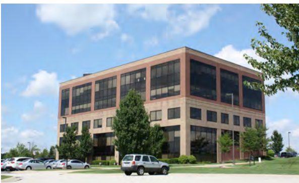
Westfield Insurance/Cisco Systems Office Building in Stonegate
