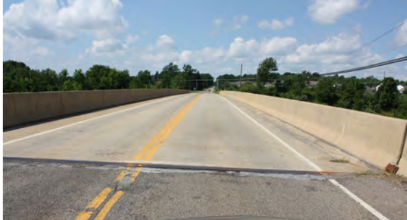
Broadview Road Bridge over I-271
