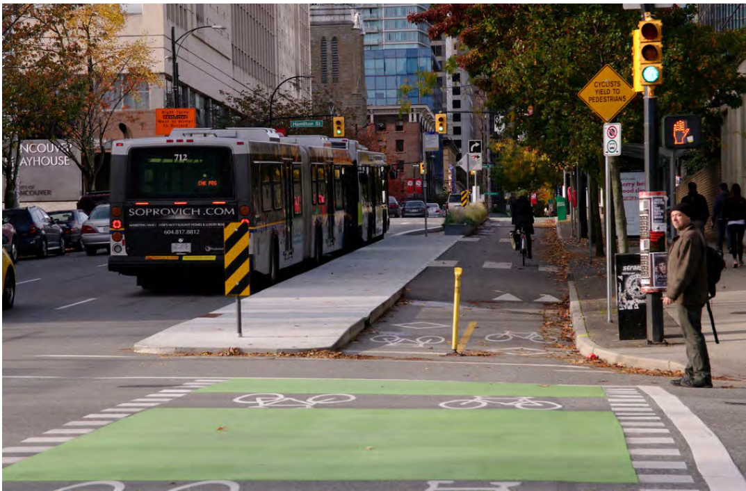
Bus stops on 2-way bike path, Dunsmuir Street, downtown Vancouver, Canada
