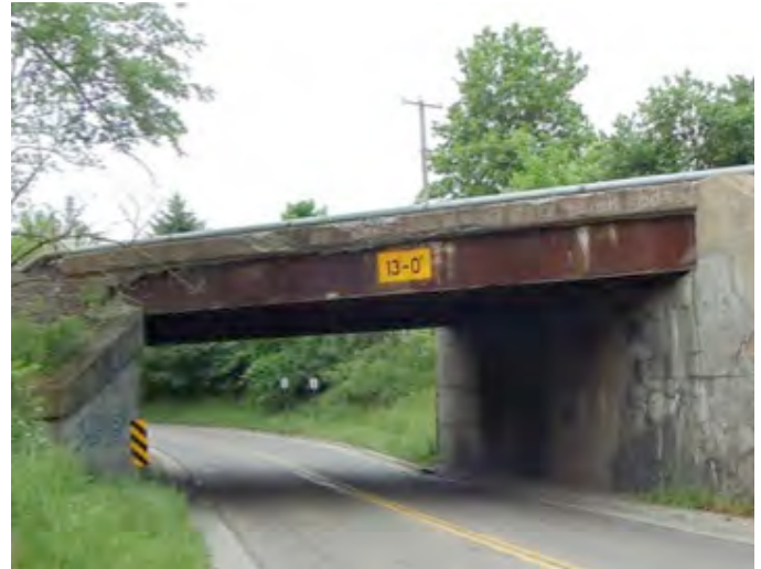
Figure 18 - Existing Railroad Bridge
