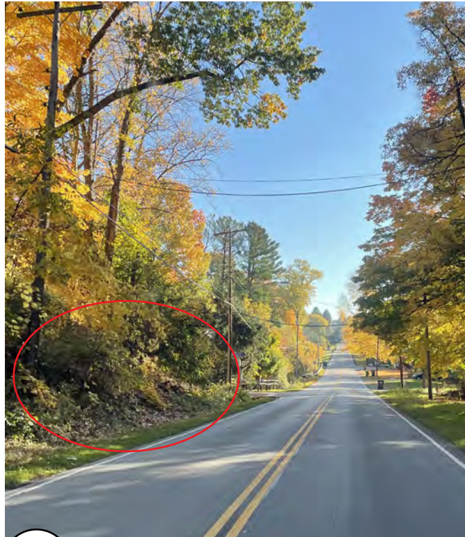
2 Existing Grades: The north side has some locations where a retaining wall or extensive grading would be needed to accommodate walks
