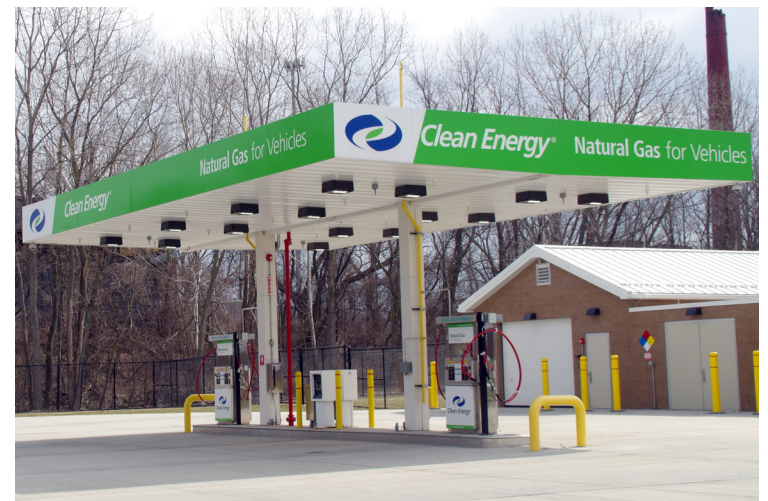
METRO CNG Fueling Station
