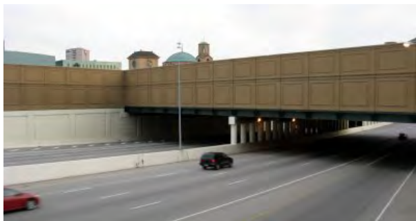
View of back side of development
