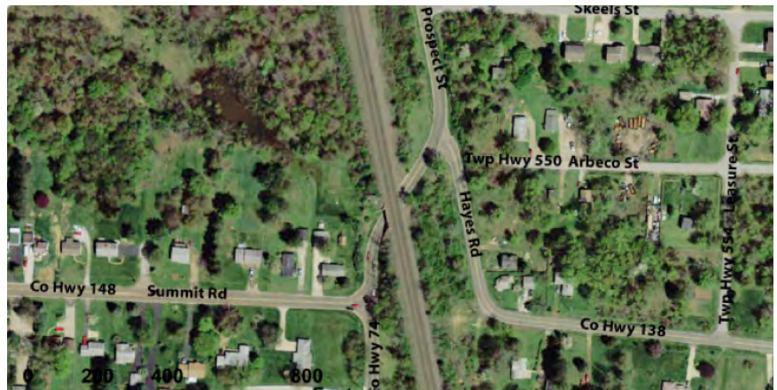
Figure 16 - Aerial View of “S” Curve - Placeholder
