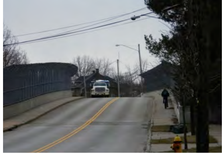
Figure 21: Existing Southerly Gateway over the CSX Railroad
