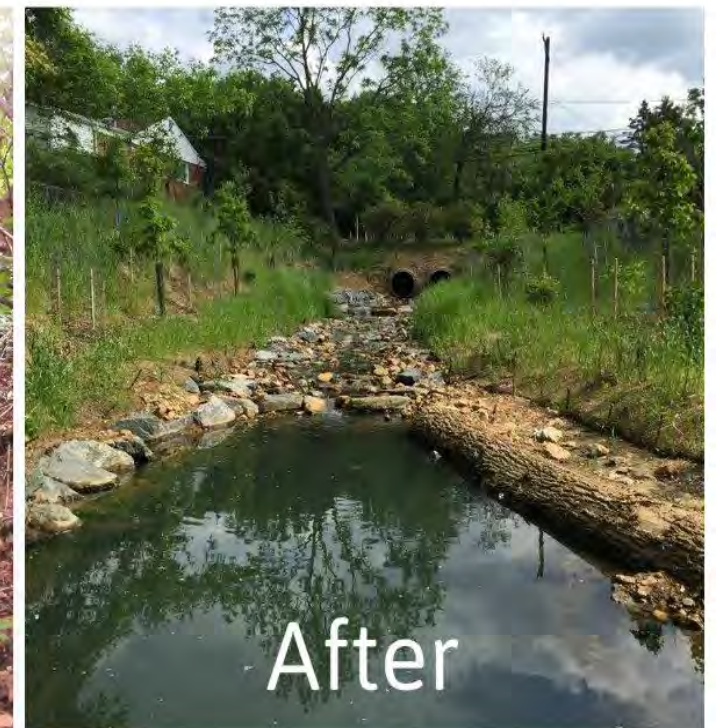
Photo 6 & 7: Photos illustrating one type of natural streambank restoration technique. Streambanks are laid back to provide storage during flooding, native vegetation is planted for shading and toe rock is installed for erosion armoring
