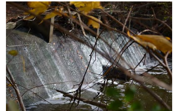
Photo 2: Mill Pond dam and underflow pipe
