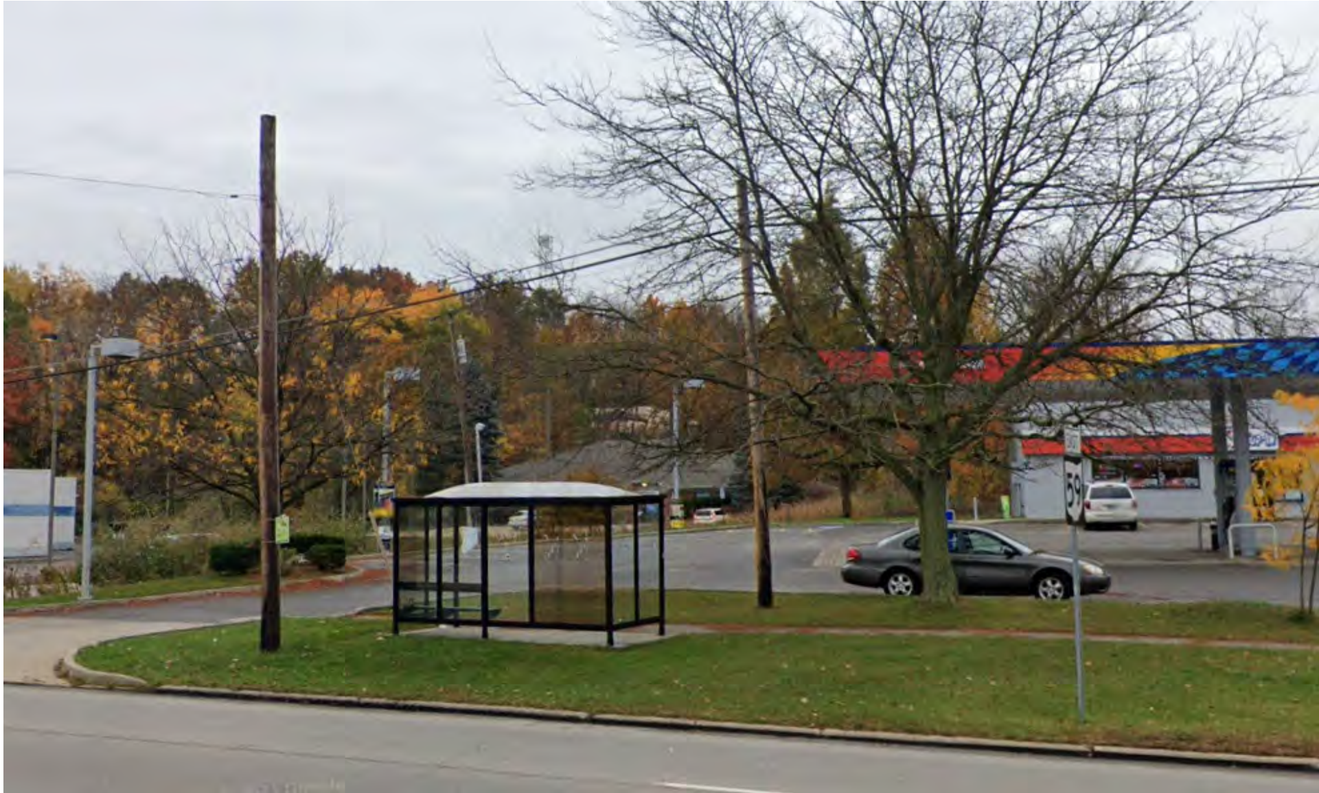
FIGURE 10 Rhodes Road bus shelter is inaccessible from the street.
