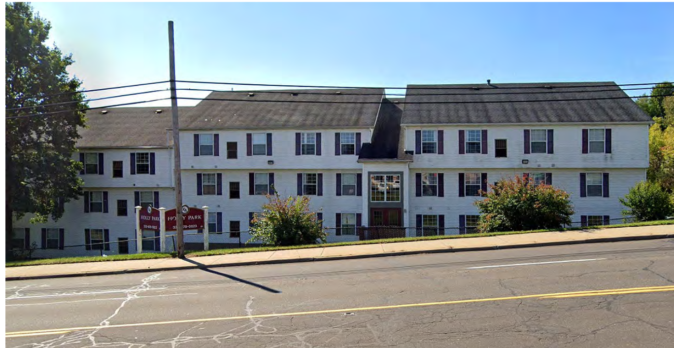
FIGURE 14 Holly Park Apartments
