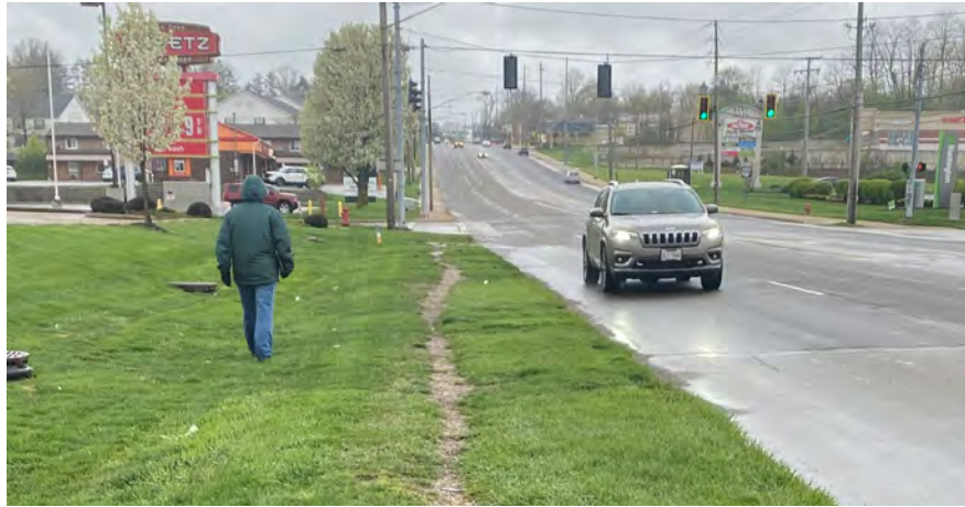
FIGURE 4 No sidewalk for pedestrians
