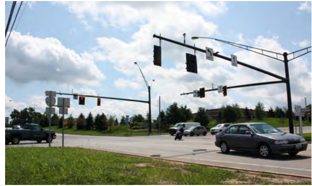
Brecksville Road - Wheatley Road Intersection
