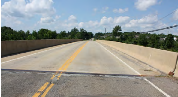
Broadview Road Bridge over I-271
