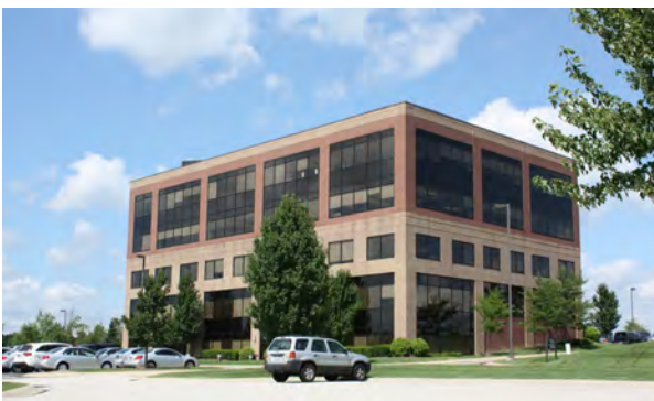
Westfield Insurance/Cisco Systems Office Building in Stonegate
