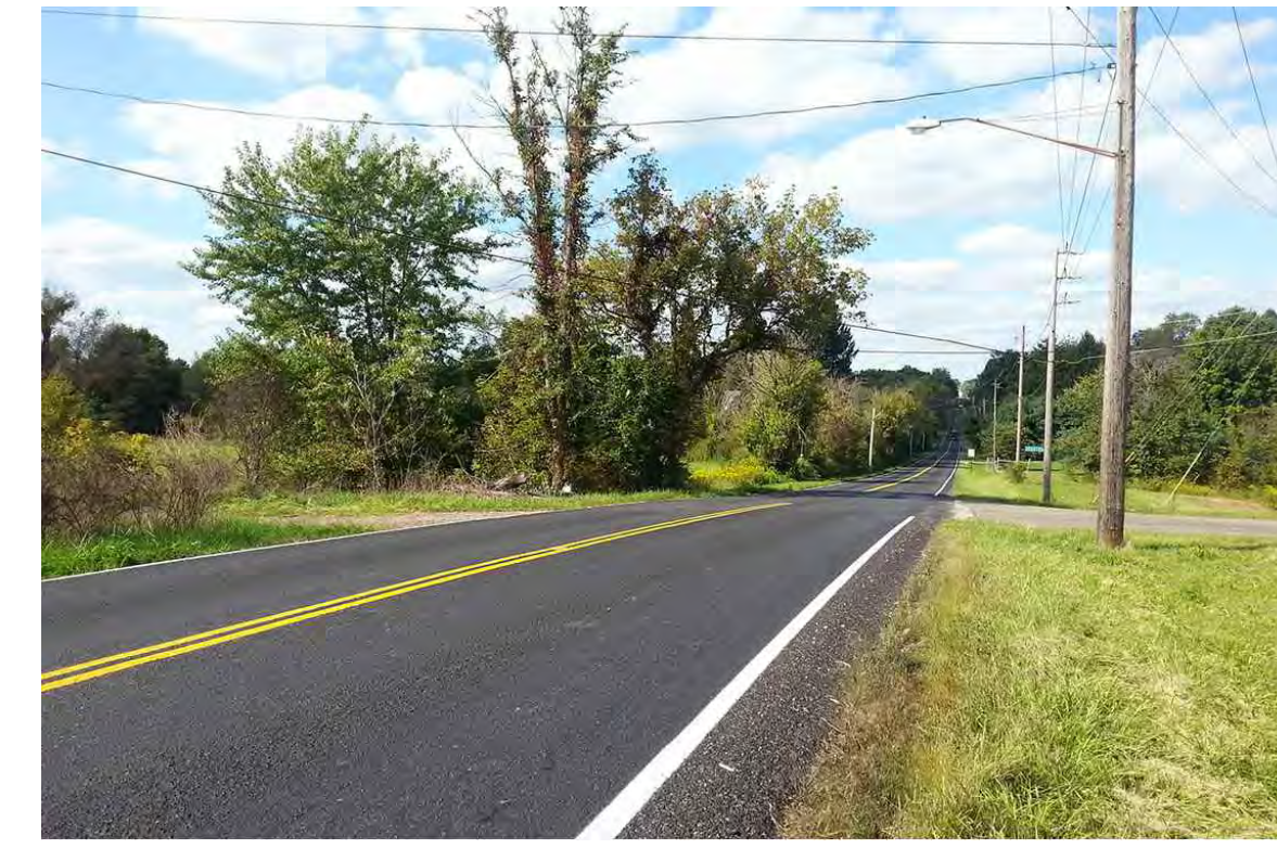
2 TRAIL CROSSING AT HAMETOWN ROAD.
