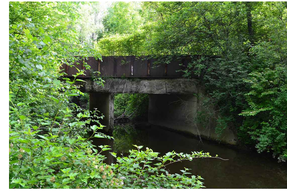
4 EXISTING INTERURBAN BRIDGE TO BE RECONDITIONED FOR TRAIL USE.
