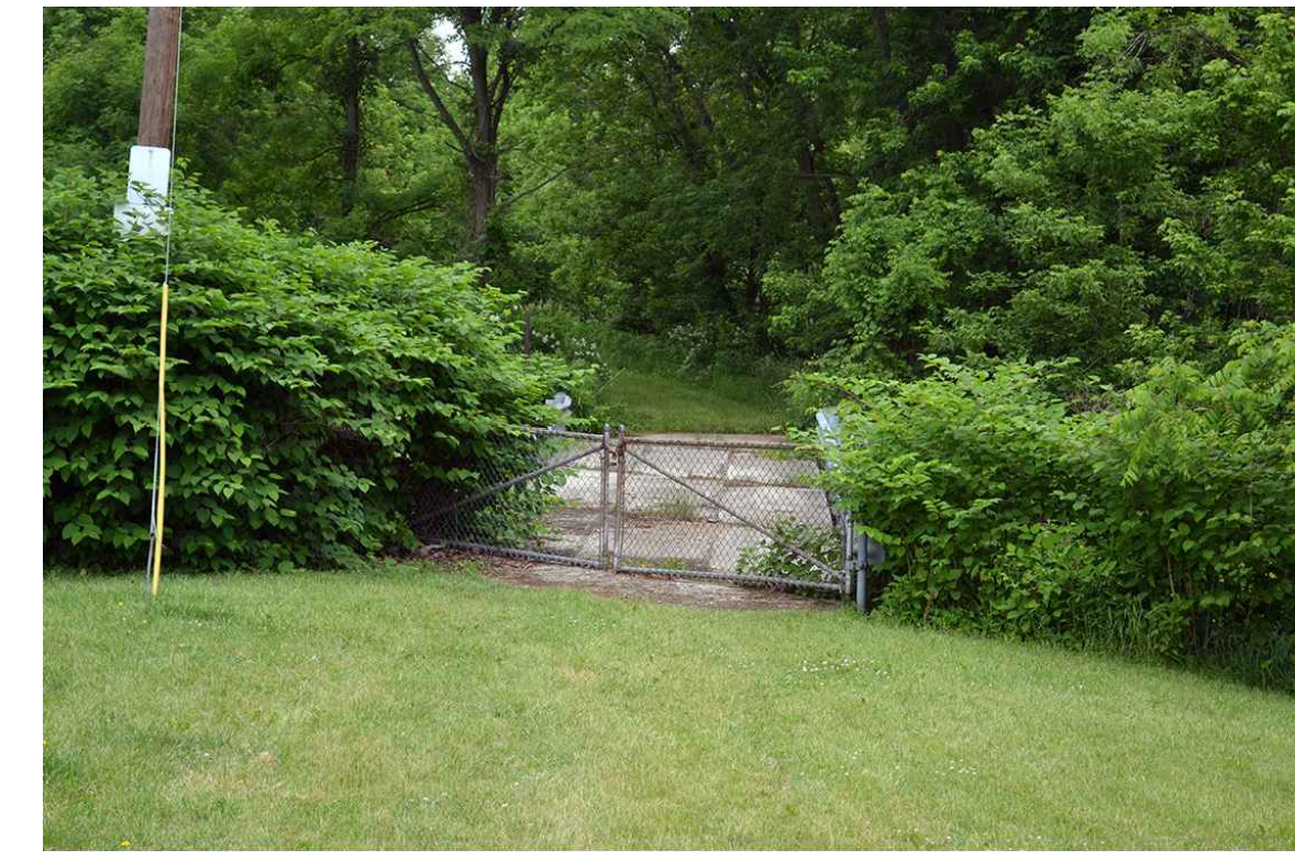
1 EXISTING MAINTENANCE BRIDGE AT WOLF CREEK.
