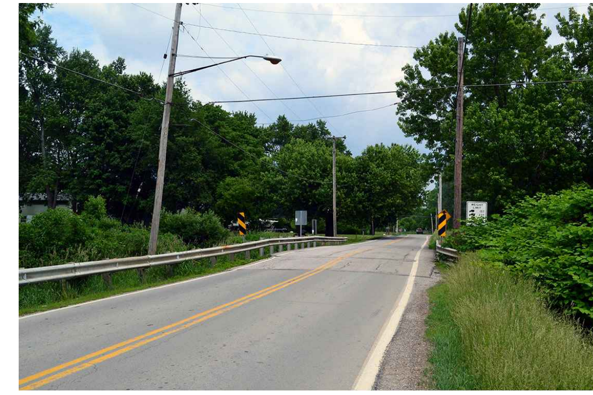
2 EXISTING BRIDGE ON WRIGHT ROAD.
