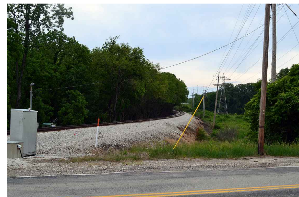
1 TRAIL TO BE DEVELOPED IN POWER LINE EASEMENT ADJACENT TO RAILROAD RIGHT-OF-WAY.
