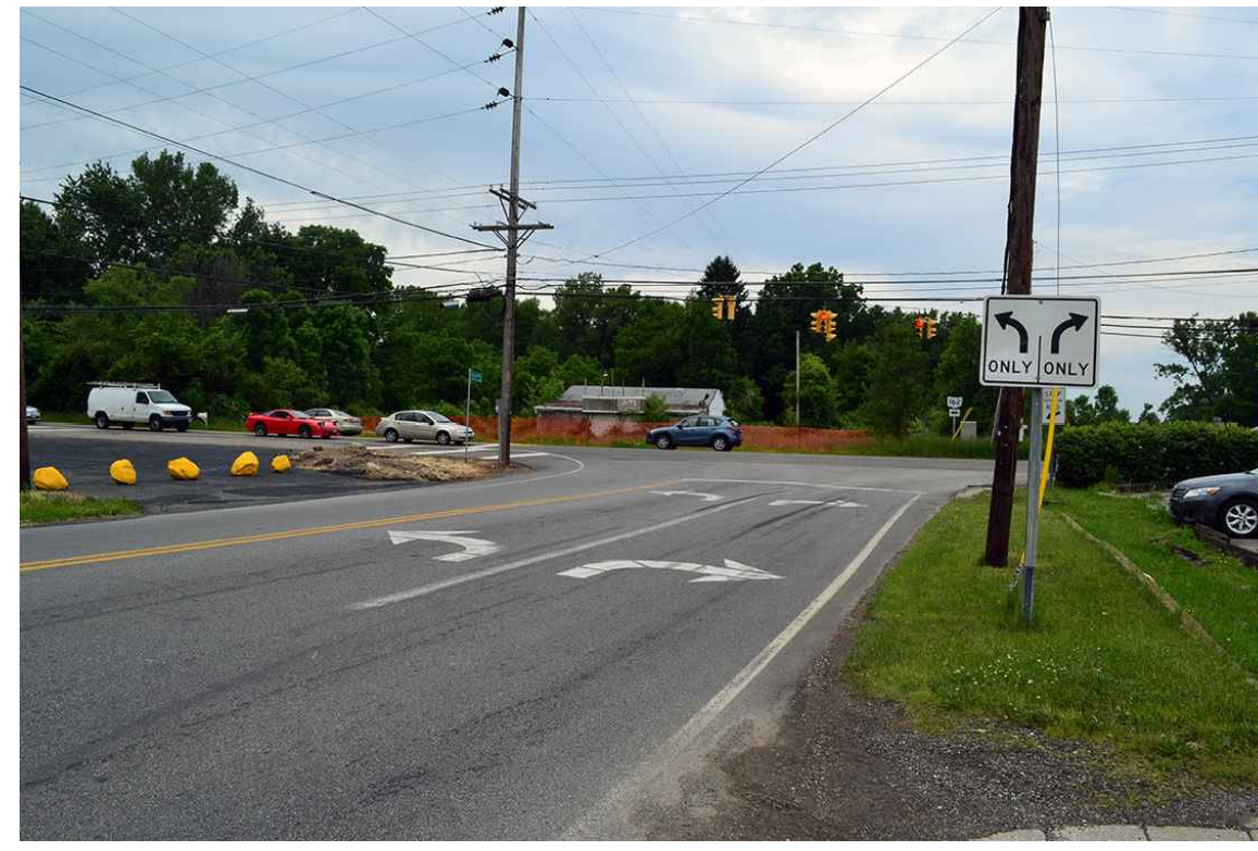
1 INTERSECTION OF COLLIER AND COPLEY ROADS. TRAIL TO UTILIZE EXISTING SIGNALIZATION WITH PROPOSED CROSSWALKS AND PEDESTRIAN ACTUATORS.
