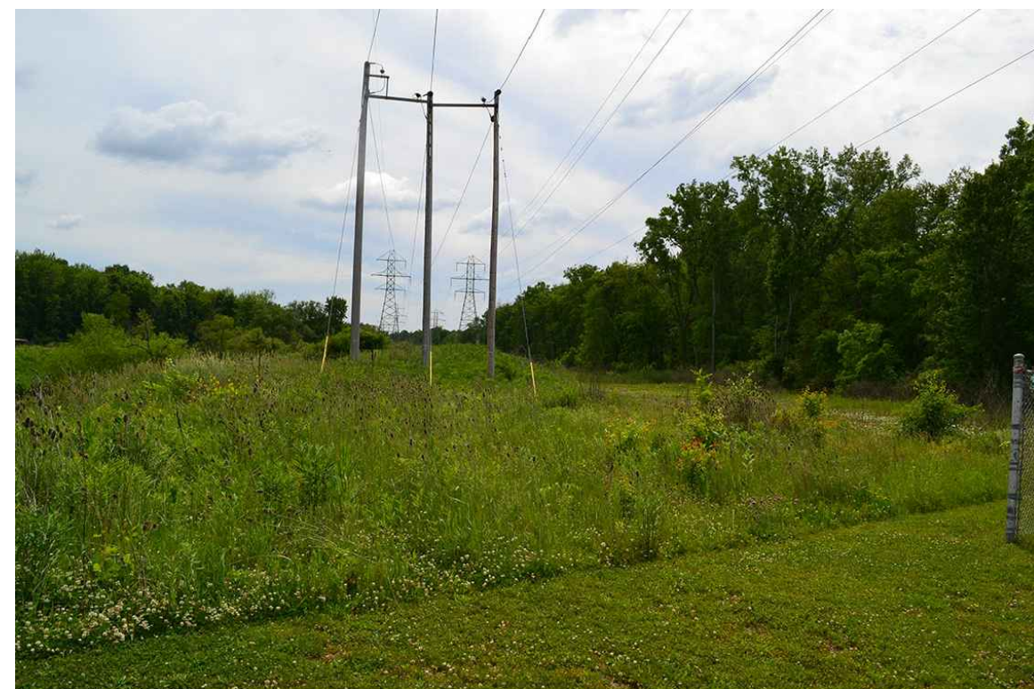
3 TRAIL TO BE DEVELOPED BENEATH EXISTING POWER LINES.
