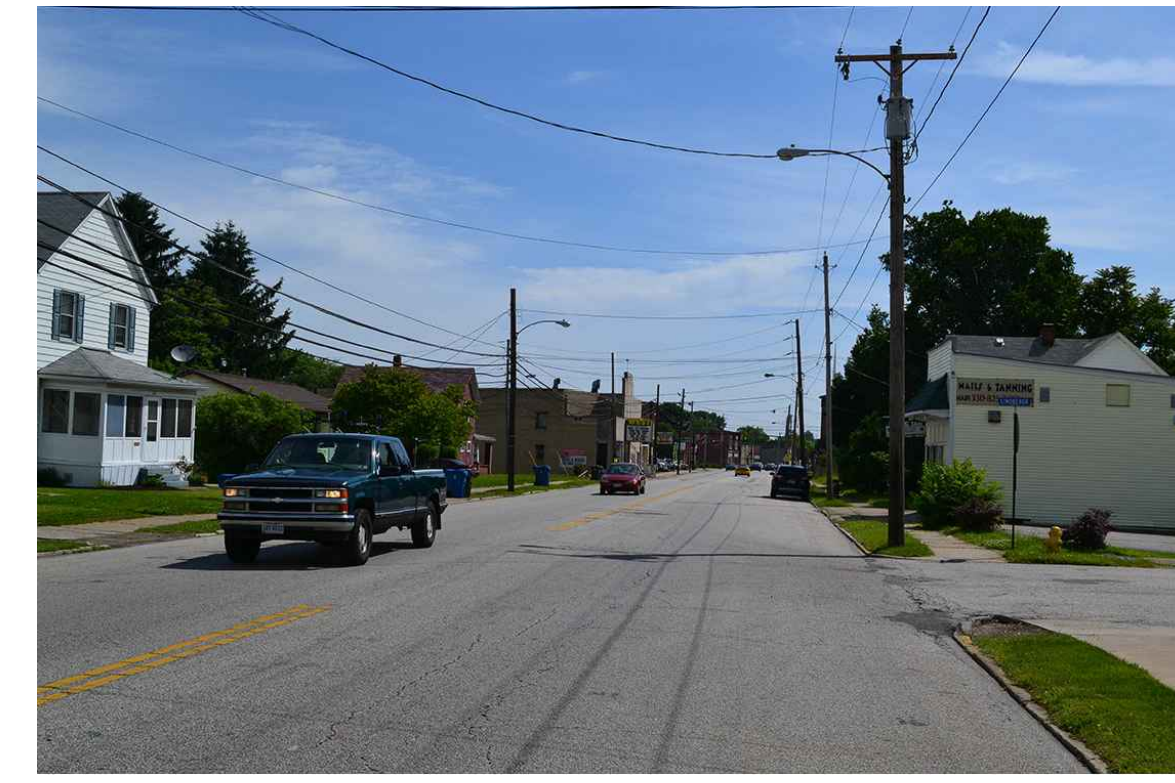
4 WOOSTER ROAD TO BE RECONFIGURED TO THREE LANES WITH A SIDEPATH ON THE NORTH (LEFT) SIDE.
