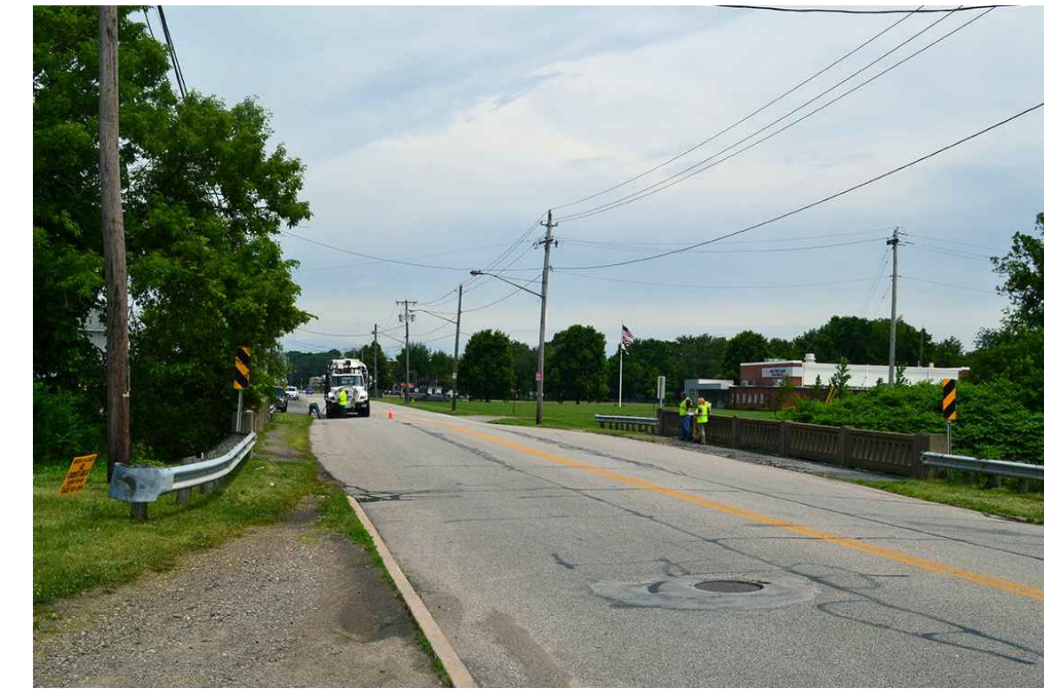
2 EXISTING BRIDGE ON NORTON AVENUE
