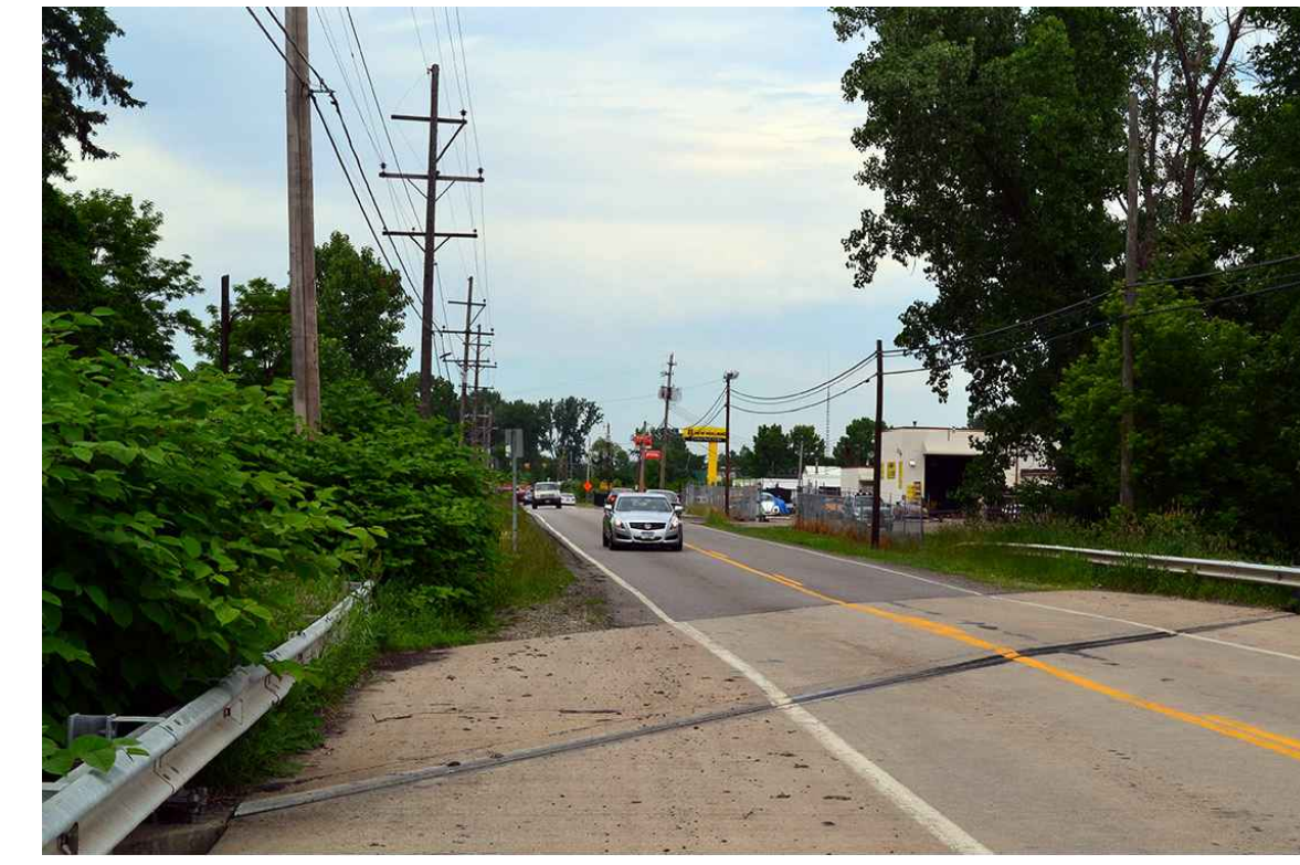
3 EXISTING BRIDGE ON COLLIER ROAD. DEVELOP SIDEPATH WITH BARRIER ON WEST (LEFT) SIDE.
