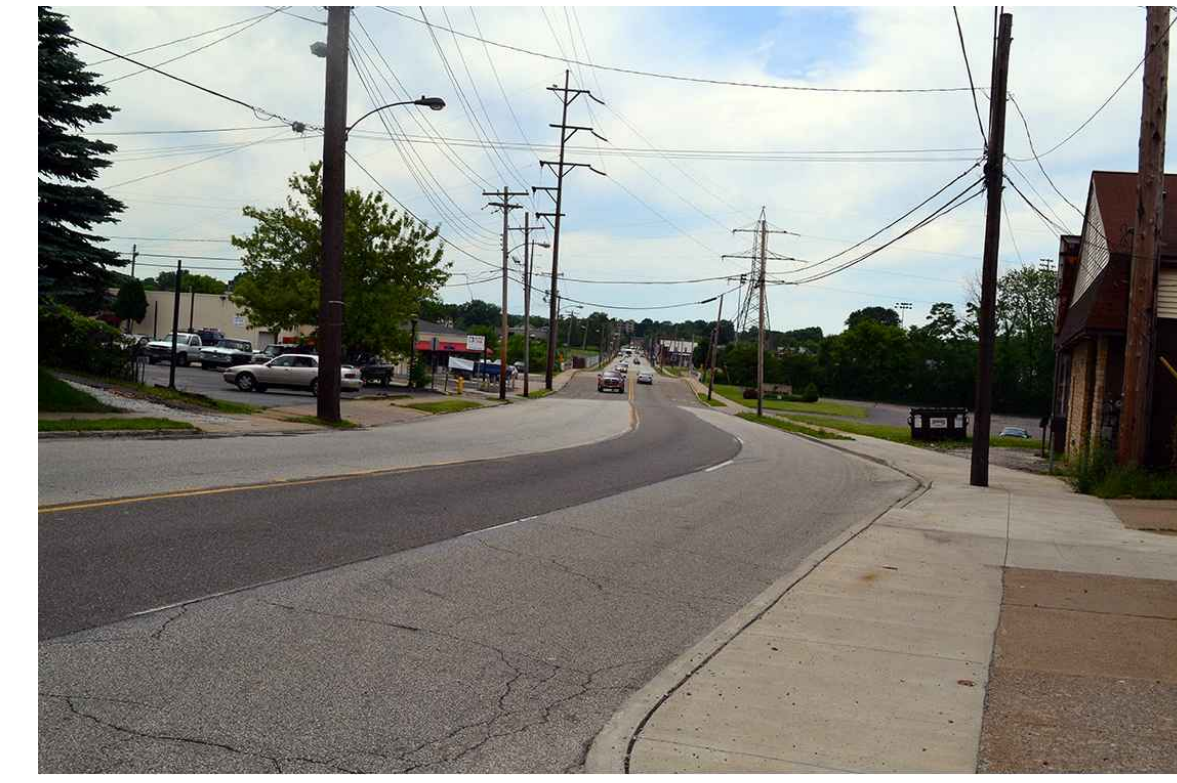
3 WOOSTER ROAD TO BE RECONFIGURED TO THREE LANES WITH A SIDEPAATH ON THE NORTH (RIGHT) SIDE.
