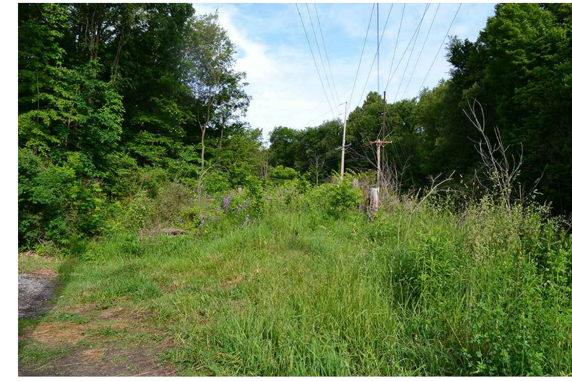
4 OVERHEAD POWER LINES ABOVE PROPOSED PEDESTRIAN BRIDGE TO BE PROTECTED DURING CONSTRUCTION.
