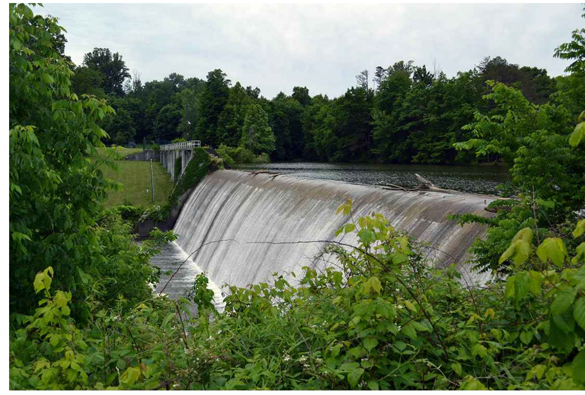
1 EXISTING BARBERTON RESERVOIR DAM.
