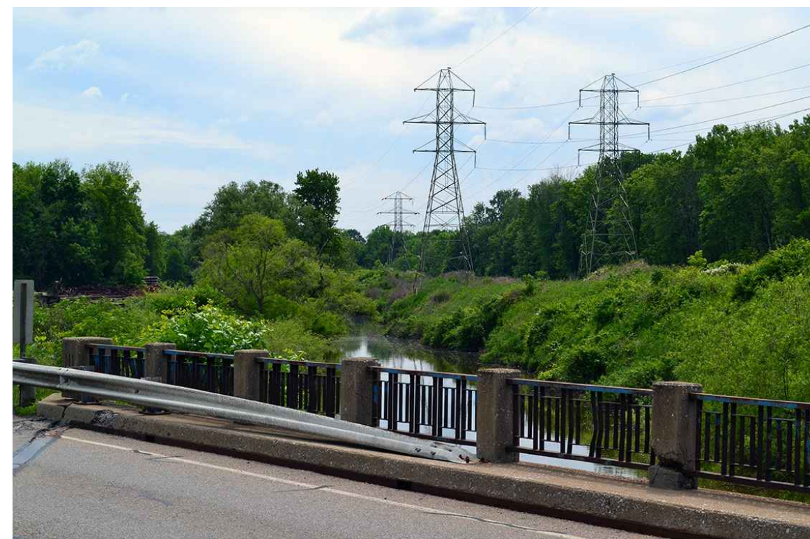
2 EXISTING BRIDGE ON BARBER ROAD LOOKING TOWARD PROPOSED PEDESTRIAN BRIDGE LOCATION.
