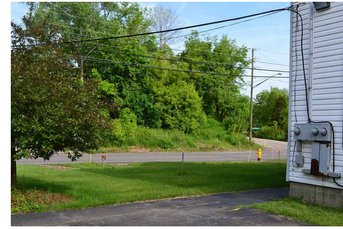
2 PROPOSED ROAD CROSSING AT 31ST STREET. REGRADE EXISTING EMBANKMENT TO ALLOW FOR 5% MAXIMUM TRAIL GRADE.
