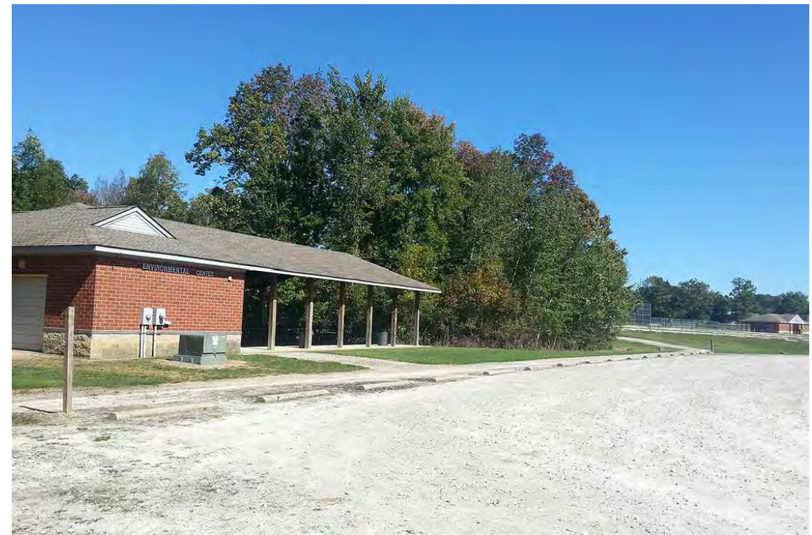
3 REFINE/REGRADE EXISTING PATH FOR TRAIL USE.
