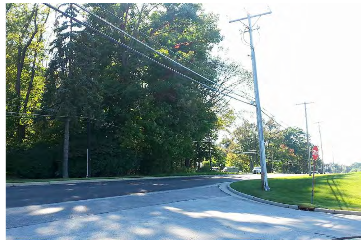
2 TRAIL CROSSING AT POTENTIAL FUTURE SIGNALIZED INTERSECTION WITH A BRIEF SIDEPATH ON RIDGEWOOD ROAD.
