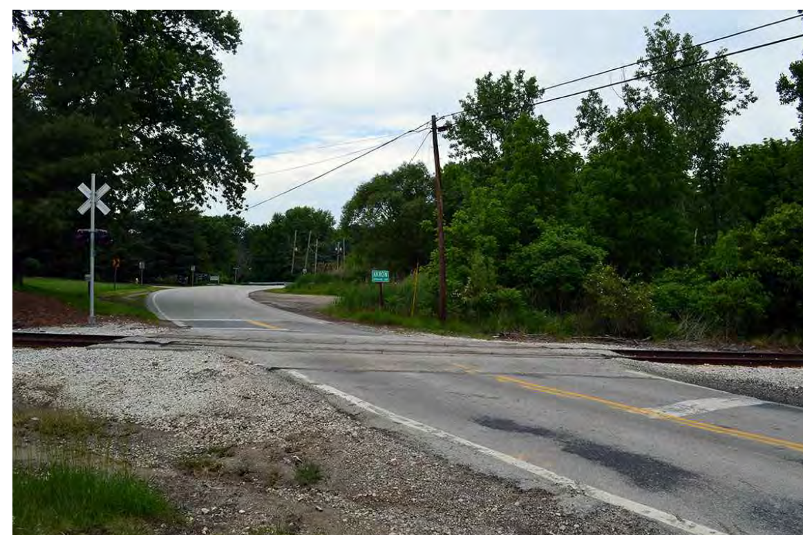
2 PROPOSED SOUTHERN TRAIL CROSSING AT SCHOCALOG ROAD TO UTILIZE EXISTING RAIL CROSSING.
