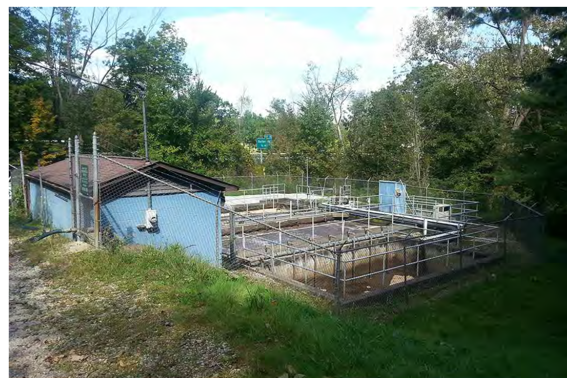
2 WASTE WATER TREATMENT PLANT PLANNED FOR FUTURE DEMOLITION.
