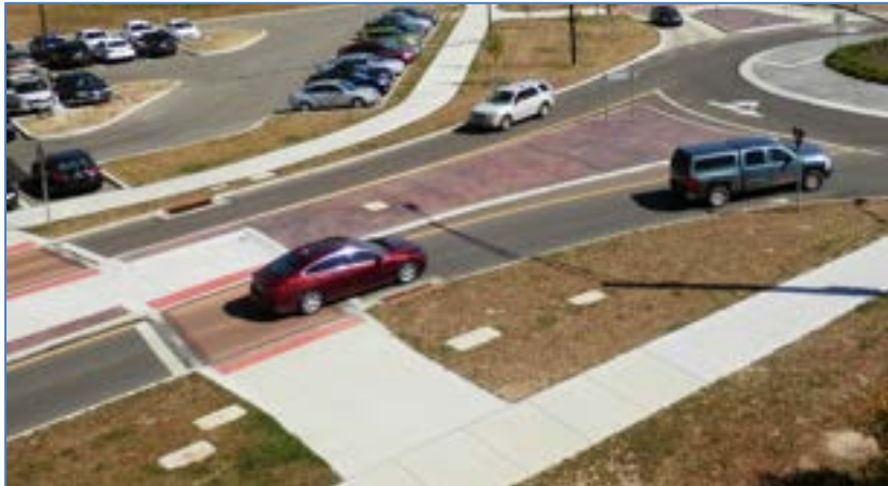
When the City of Kent constructed this roundabout on Summit Street, the crosswalks were staggered. Placing crosswalks further from exiting traffic reduces chances for conflict.
